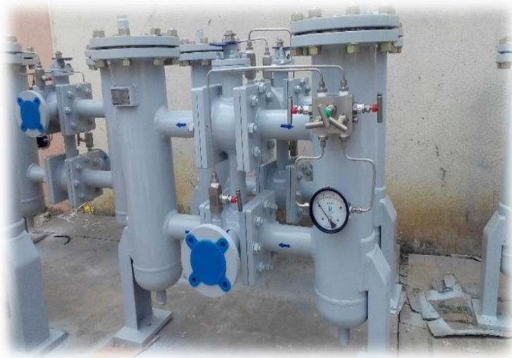
2½" DUPLEX STRAINER ISOLATION WITH 6WAY DIVERTOR VALVES
